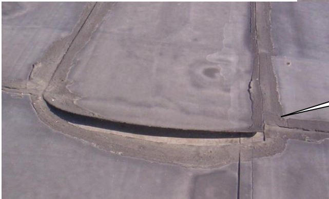
Typical field seam that is loose, but not leaking
